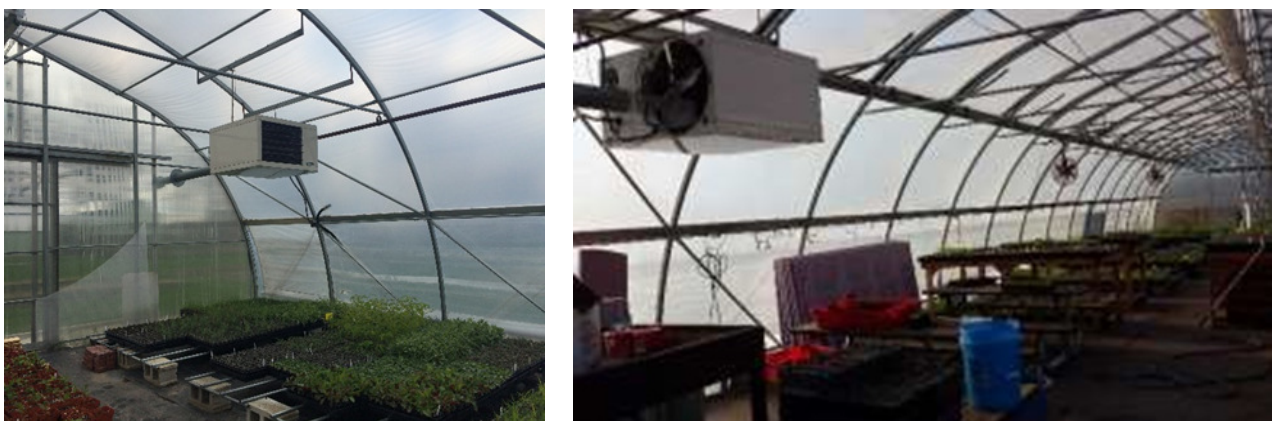
Figure 4: Location of heaters inside the greenhouse (Source: J.C Reuthinger Preserve, Oregon Road,OH)
